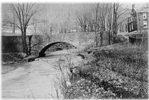
Built in 1841, the stone bridge over Little Sewickley Creek was enlarged in 1918 and remains in use. The photo on the left shows the bridge as it appeared in 1905. The Little Sewickley Creek Bridge #1 is found in what is now Edgeworth Borough.
